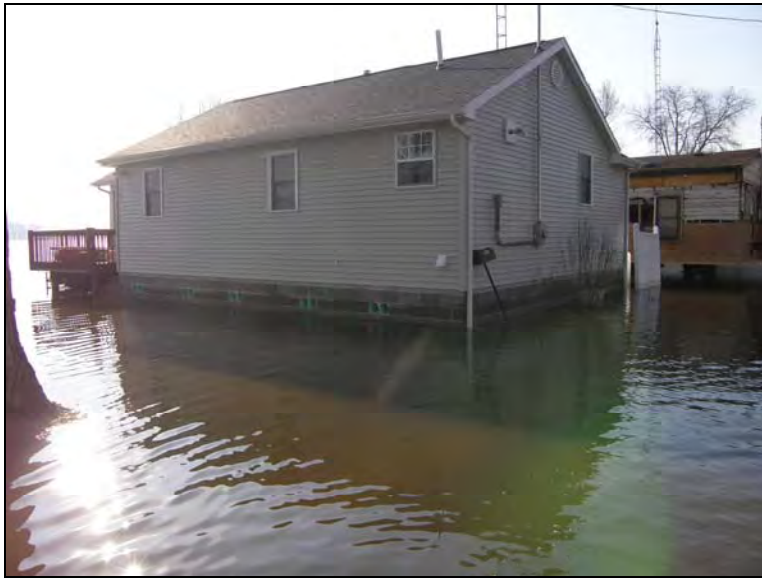
Figure 5-6. Waldron Lake – home damaged by 2008 flood repaired and elevated (enclosure beneath lowest floor with flood vents), utilizing flood insurance/ICC.
