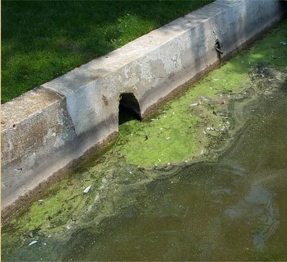
Traditional shoreline protection has relied on "hard armor" measures such as concrete seawalls, sheet pile, and rip-rap. While effective at preventing shoreline erosion, these techniques can have several detrimental effects to a lake.
